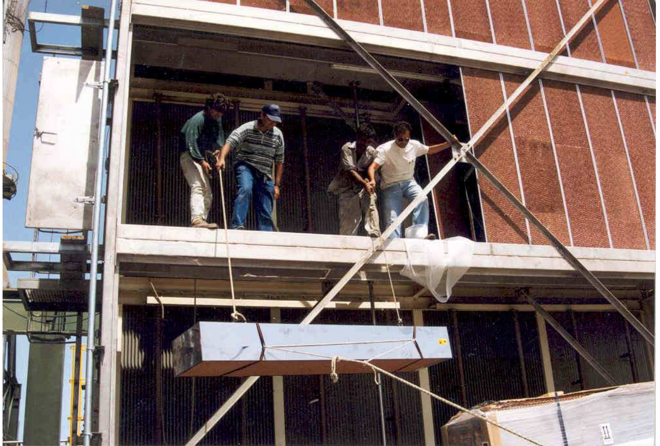
ABB gas turbine in Chania/ Greece
