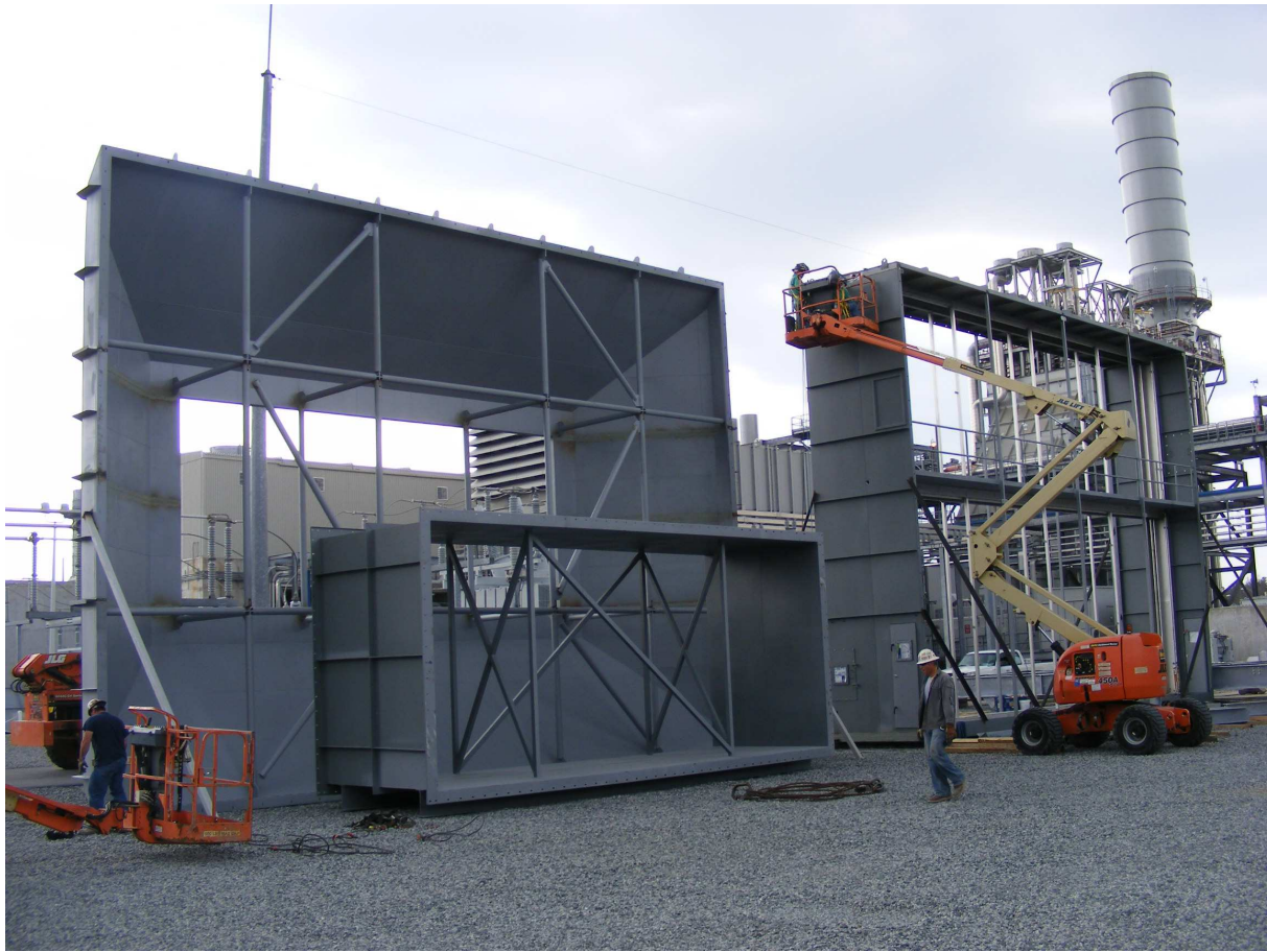
transition pieces + cooler module prior to lifting
