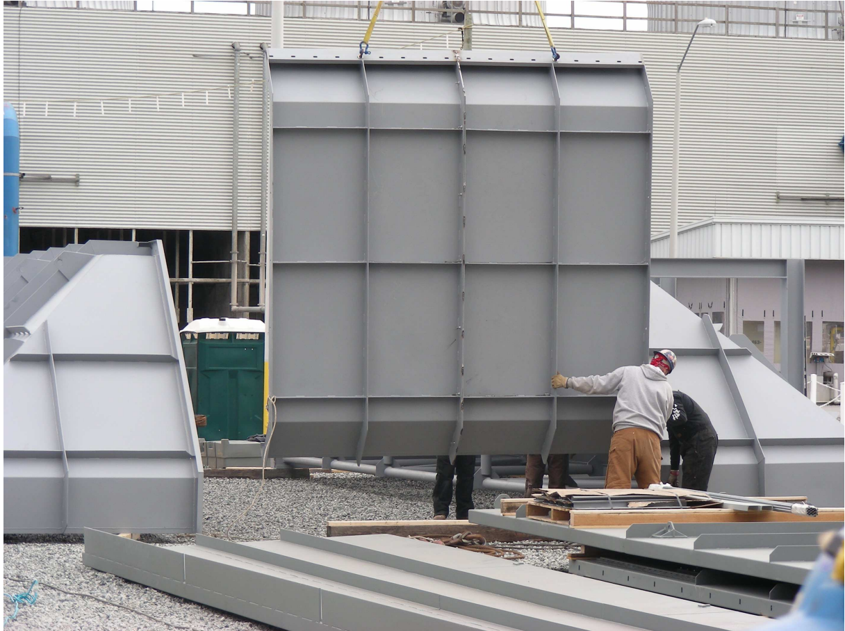
assembly of new transition piece
