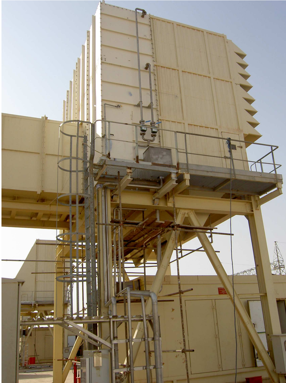
Frame 6 with new transition piece/ downstream evapcooler after installation
