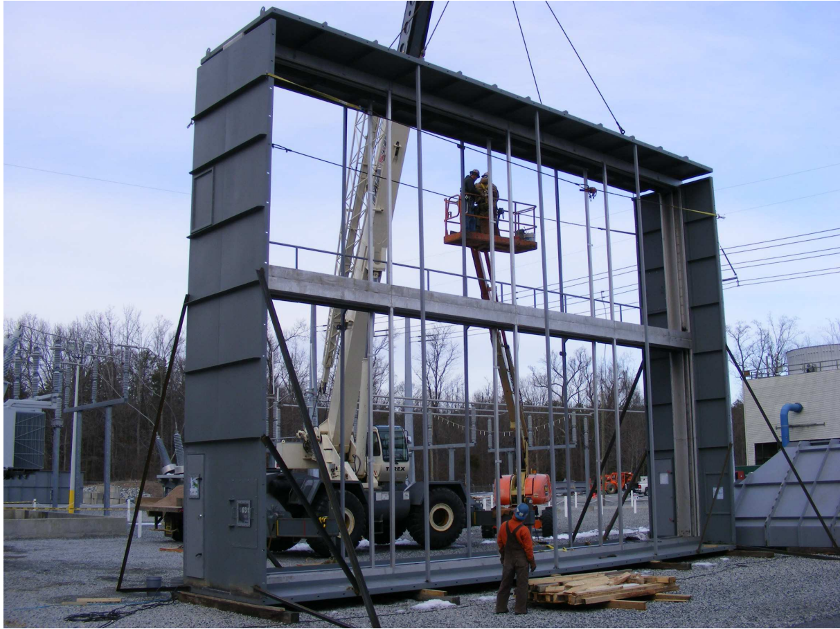
insert of stainless steel evaporative cooler into carbon steel casing with service access
