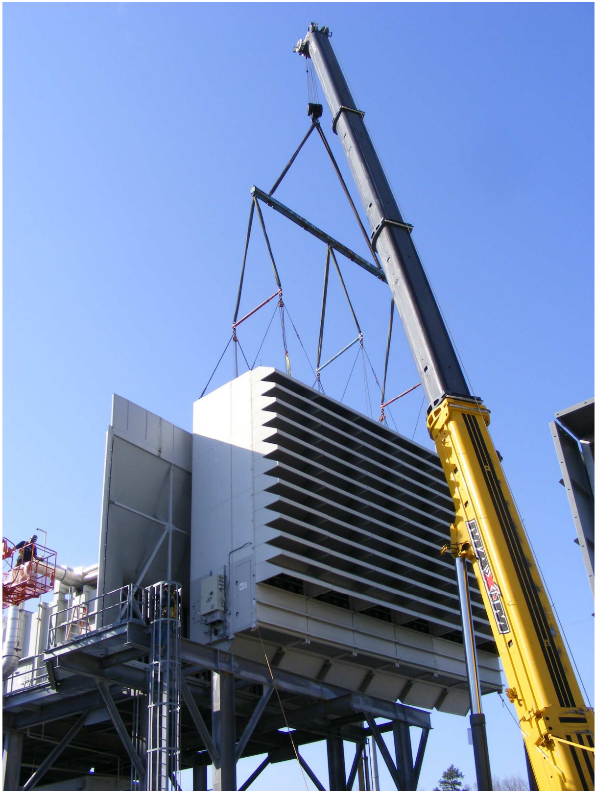
removal of existing pulsefilter housing
